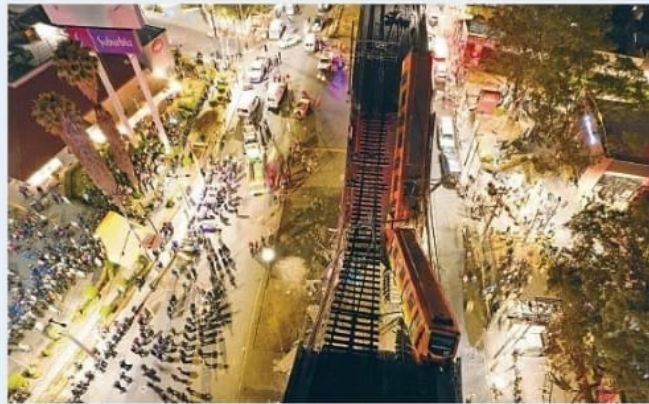
The Mexico City train overpass collapse fueled outrage and demands for a probe.
