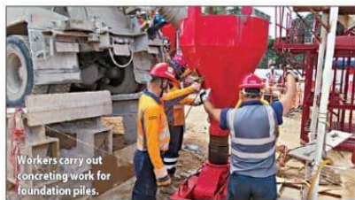
A mixer lorry unloads concrete.
