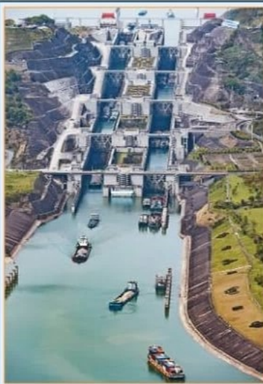
Three Gorges Dam has a locks system as well as a shiplift system.
