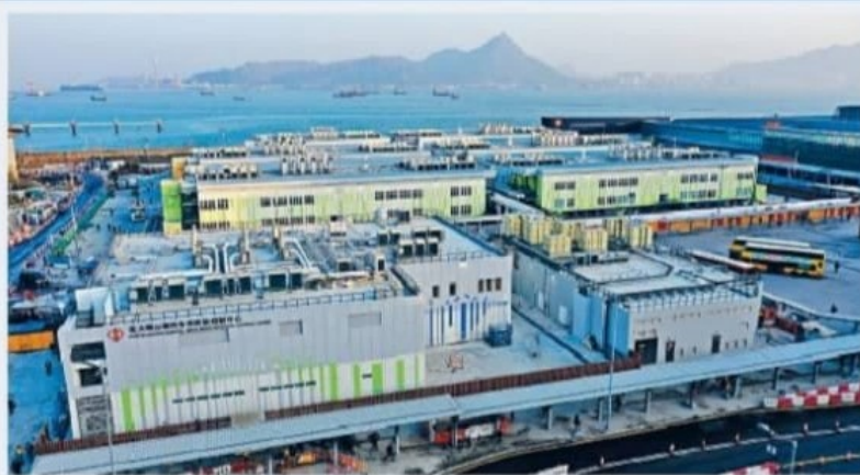
The Hong Kong Infection Control Centre was built in just four months. XINHUA
