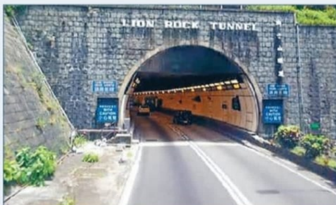
Lion Rock Tunnel is an example of a drill and blast tunnel.
