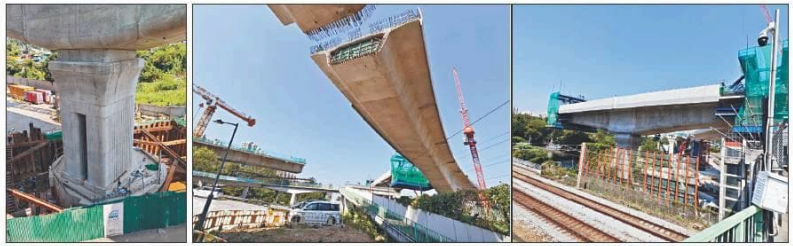
Clockwise from above left: the column holding up the long 120-meter viaduct section with the bearing concreted up; the section to be rotated into place; the viaduct section that needs to be joined up with adjacent sections; and the bypass site with its attendant complications with East Rail tracks, high-voltage underground lines and water mains nearby.
