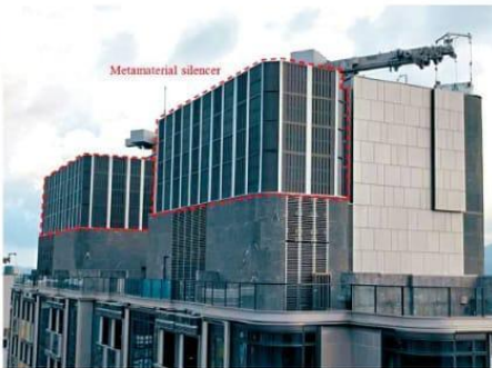
The interlacing air pockets in the layers of plastics work in unison with the plastic layer to form a composite panel with much more effective sound absorption.
